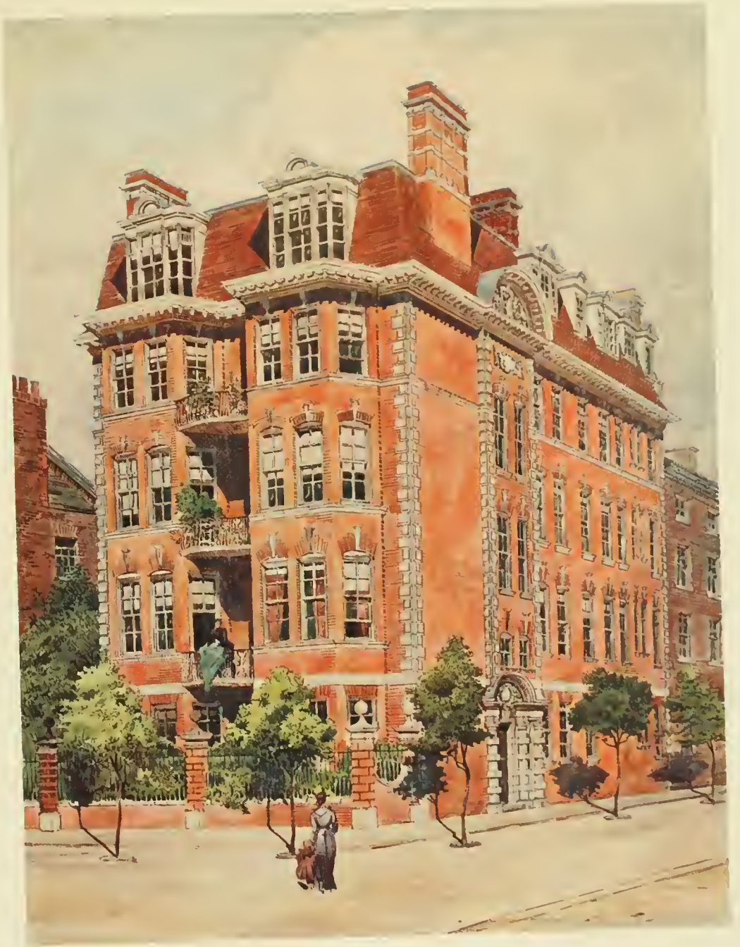
BLOCK OF FLATS, EARL'S COURT SQUARE, LONDON. MATERIALS - RED FACING BRICKS, BATH STONE DRESSINGS; THE ROOF COVERED WITH TILES, THE WOODWORK PAINTED WHITE.
